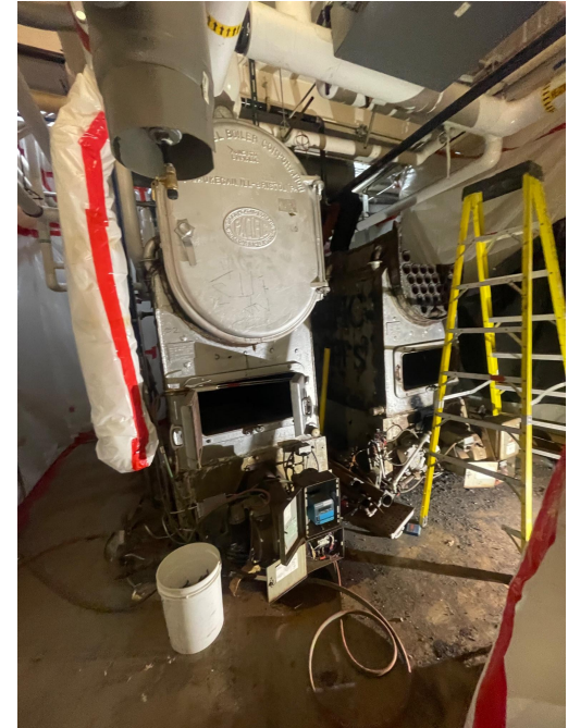
Old boiler demolition
